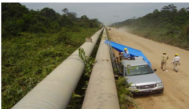
Fig. 1. Radiotracer experiment on multiphase flow in the HCT pipeline.
